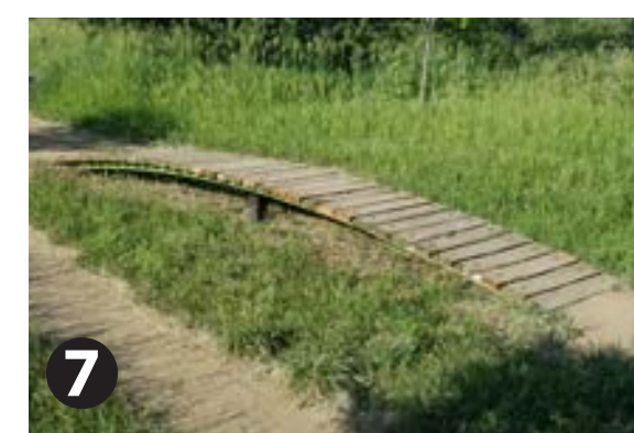
30' wide wood bridge, max. height of 18" in the center
