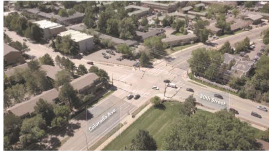
EXISTING CONDITIONS - LOOKING SOUTHWEST
