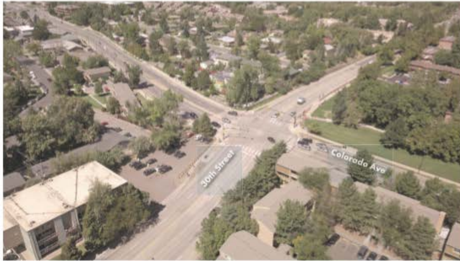
EXISTING CONDITIONS - LOOKING NORTHWEST
